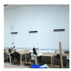
2/3 Ceramicx FTF Ceramic Flements IR2 Heater size 509 x 100 x 166mm - 3.4kg IR3 Heater size 760 x 100 x 166mm - 4.4kg Aluminised steel reflectors Heating Up Time < 5 Minutes Useful Wavelength Range 2 - 10 µm IP rating: IPX4
